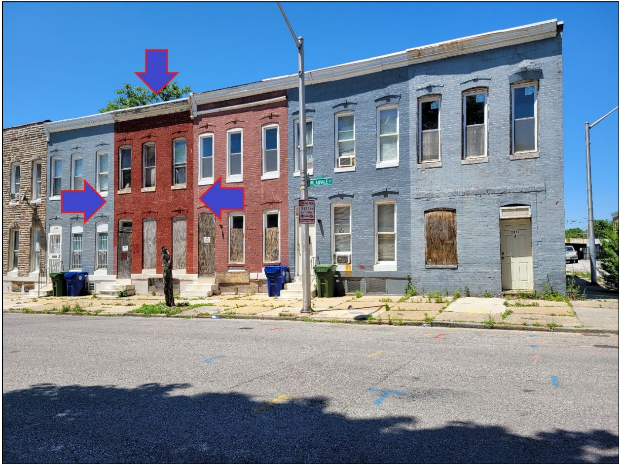
2) Front view of Subject. Picture taken facing north.
